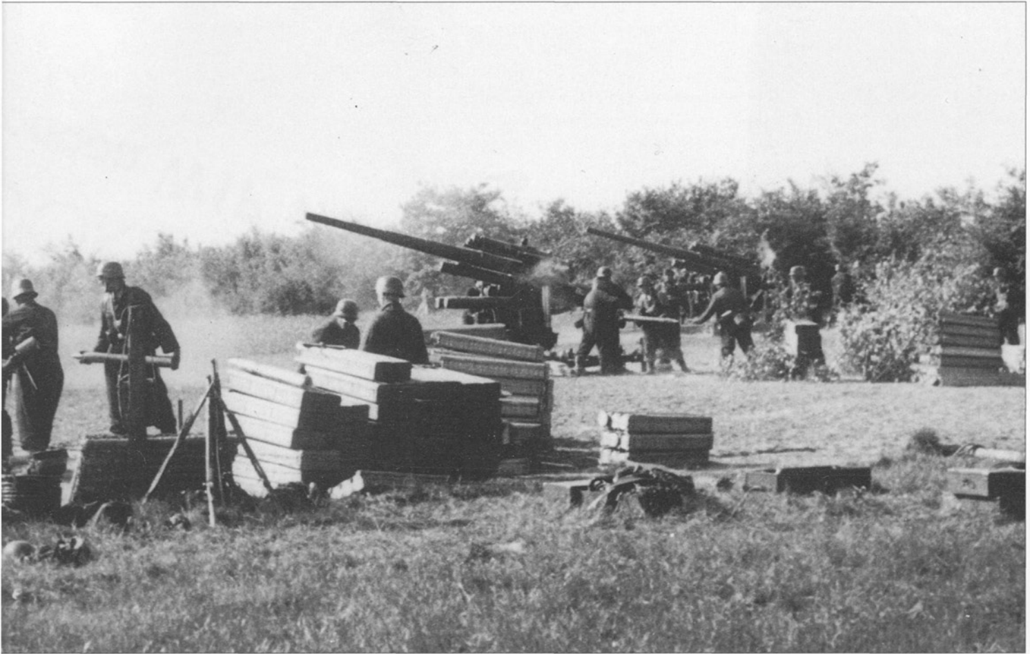
ABOVE German anti-aircraft artillery in action. The German armed forces employed their 8.8cm guns with great versatility, using them against ground targets when necessary. They were found to be particularly effective against tanks, whose armour was too thick for conventional anti-tank guns.
